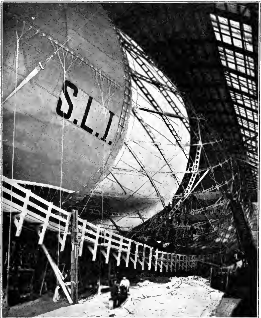
A GERMAN AIRSHIP IN COURSE OF CONSTRUCTION.
